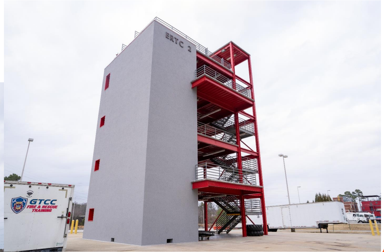
Repaired Stair Tower – Jamestown Campus
