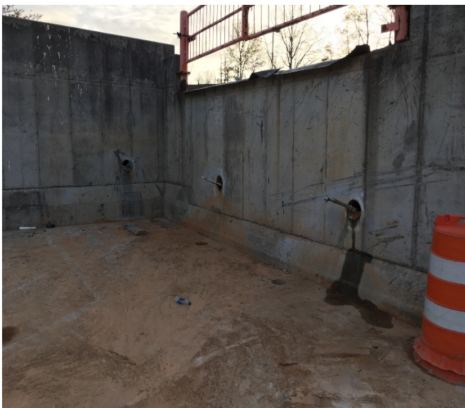
Photo No. 1 - Sample Cores Drilled into Wall
