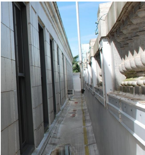
The 4th floor catwalk is covered with a TPO membrane that is generally in good condition, but is creating problems as it extends up the back of the parapet walls and is trapping moisture inside the wall. This moisture is contributing to the deterioration of the parapet. The membrane should to be removed from the wall and the brick should be cleaned of adhesive and repointed.
