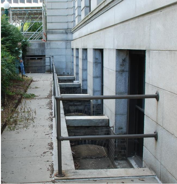
Pipe guardrails at the basement window wells.
