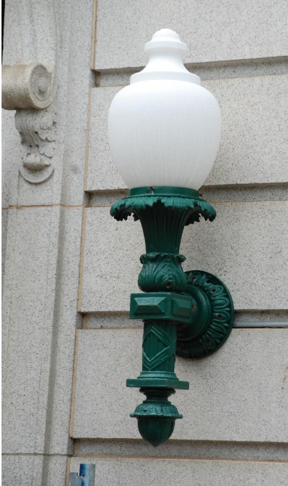
Original wall light from one of the side entrances, now relocated at the South entrance. The globe has been replaced and it was originally painted the same color as the windows and the doors.
