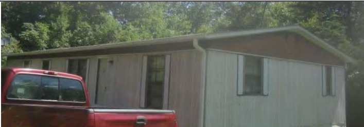
1977 – Mid-80's “aluminum” Base Grade D+ Functional Dep 5% - 15%
