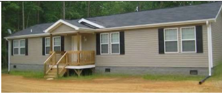
1995 – Present “modern” Base Grade C Functional Dep 0%
