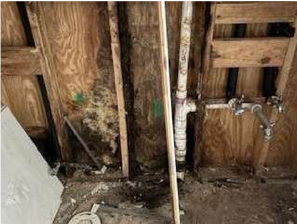
Photograph 3 – Photograph of fungal growth in a bathroom.
