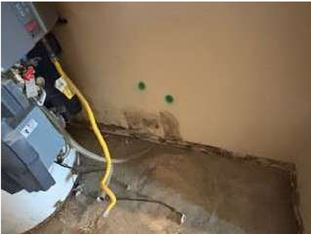
Photograph 2 – Photograph of fungal growth at water heater.
