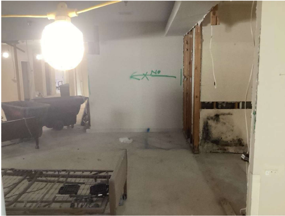
Examples of Mold Growth and Rotted Framing
