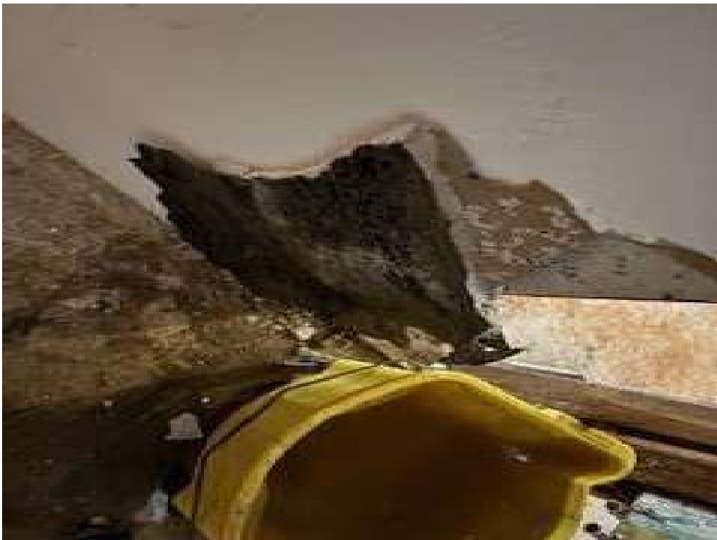
Photograph 4 – Photograph of fungal growth near a leaky pipe.
