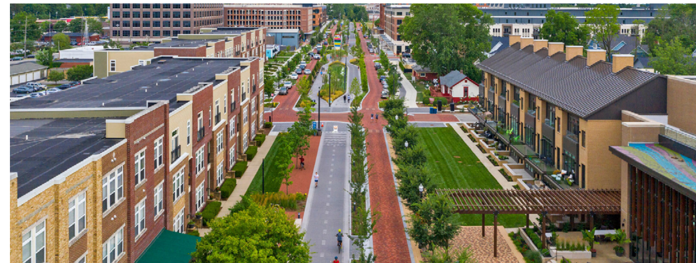
A reimagined boulevard in Carmel, Indiana provides multimodal connectivity and environmental resilience. Photo source: Landscape Performance Series, Landscape Architecture Foundation
